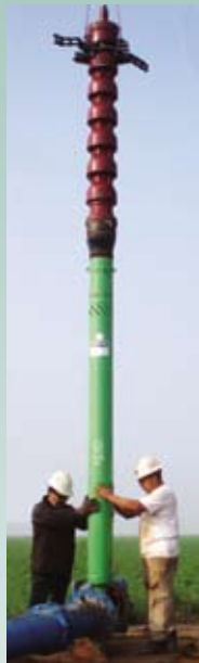
PPS During Installation
